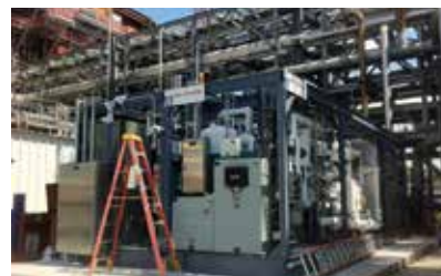
A real-world tested technology to capture CO 2 from power plants or industrial sources.
