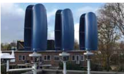
Small wind turbines suitable for urban settings, combining efficiency, low noise and synergistic clustering.
