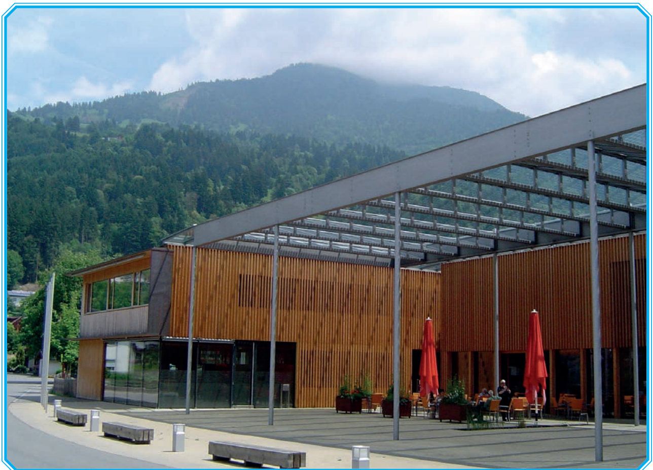
Picture 16: Ludesch Community Centre (Austria) in a passive energy standard and with a facade made of wood obtained from the surrounding forests
