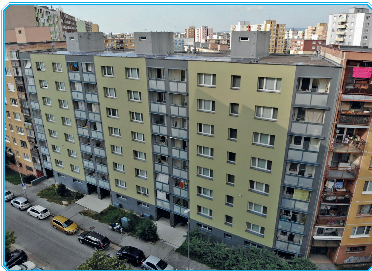
Picture 17: Increasing thermal insulation of external cladding of an apartment building (P. Horova street, Bratislava, Slovakia)
